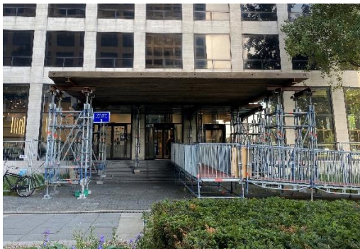
Entrance from metro station
